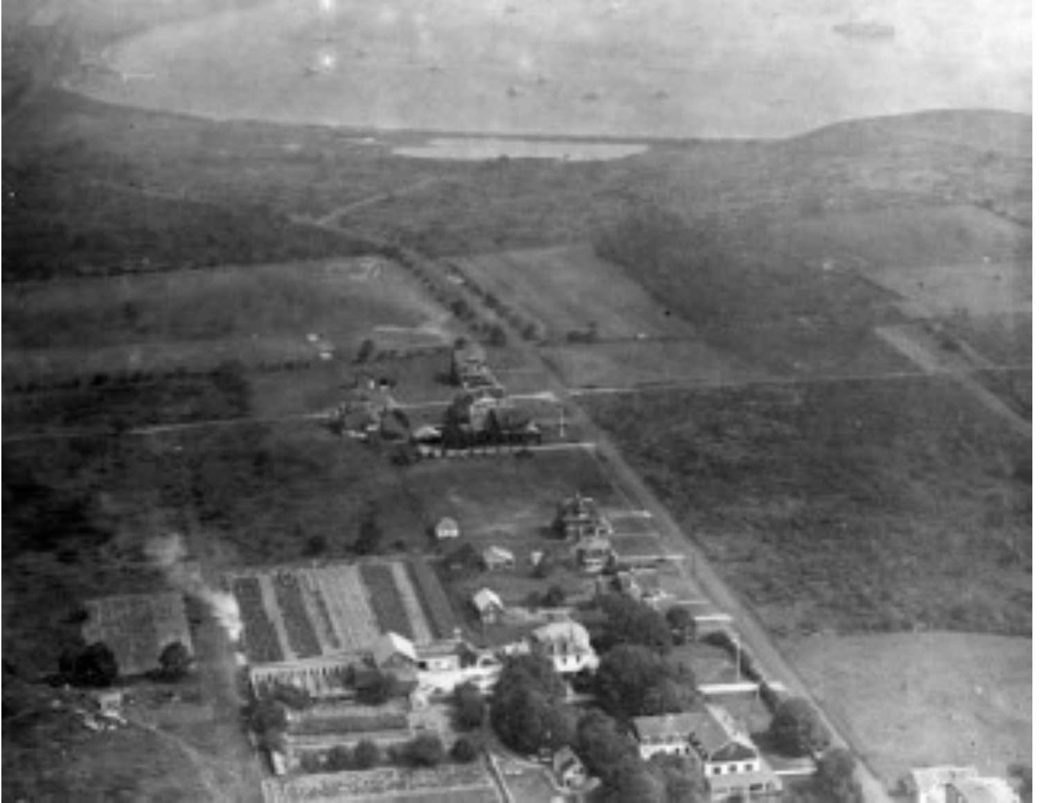
JHS photo #P2004M.400, Sanitarium 2 (Plat 8, Conanicus Ave: Aerial View, early 1920s) – “Caption: In the foreground of this photo, ca. 1920’s, is Dr. Bates Sanitarium. Going north, in the center of the picture Mt. Hope Avenue intersects with Conanicus Avenue. In the background are Freebody Pond and Potter’s Cove. Photo courtesy of F. W. Allen, Jr.” (Note: the barrier beach that formed Freebody Pond was excavated for road fill ca. 1952.)
